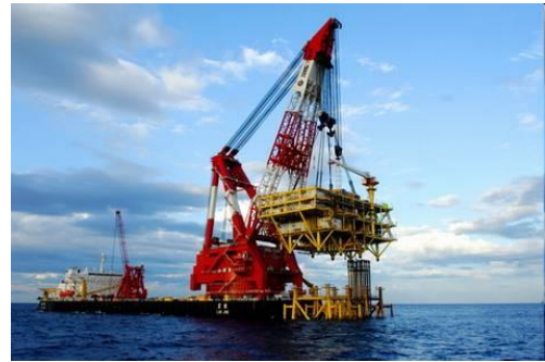
Figure 13: CNOOC floating crane
