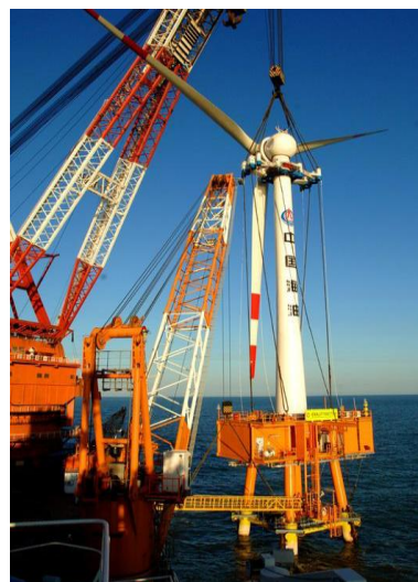
Figure 6: Bohai turbine installation Source: CNOOC
