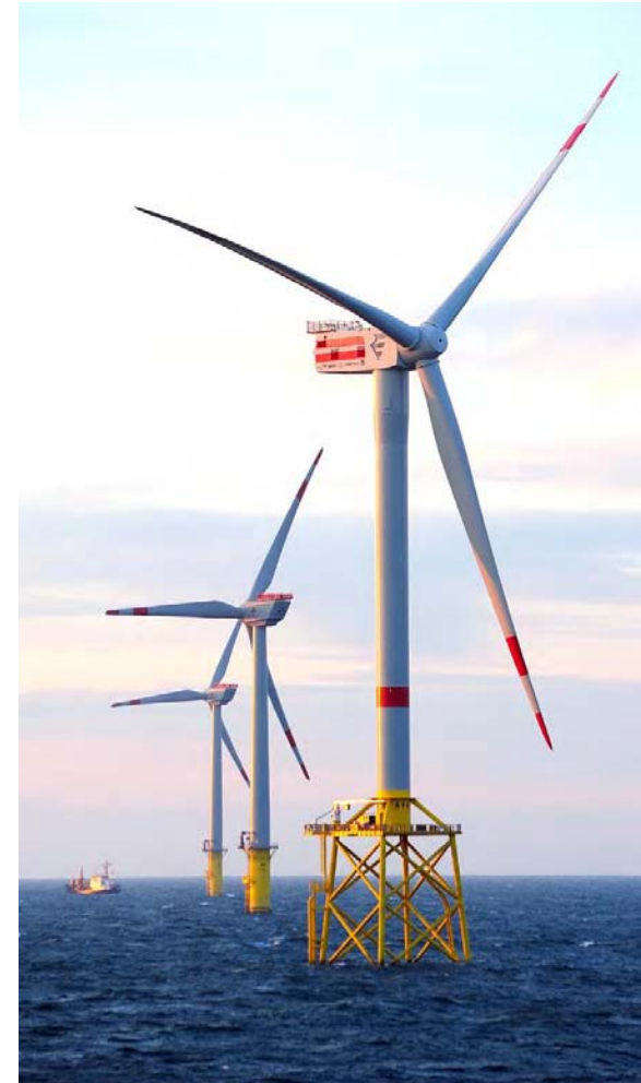
The Alpha Ventus offshore wind farm: Repower 5M on top of OWEC Tower jacket foundations in the foreground & Areva Multibrid 5M on top of Aker Verdal tripods in the background.
